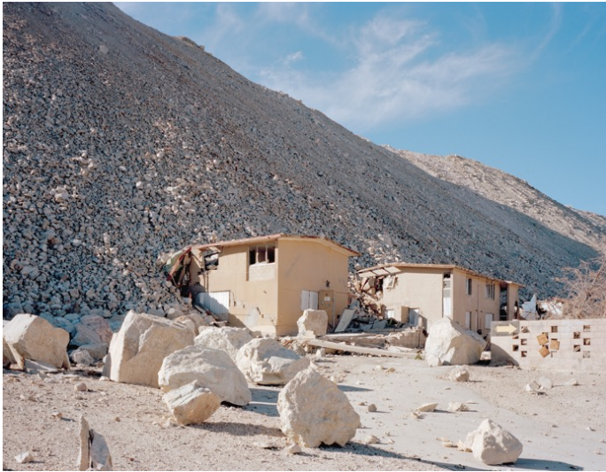
Fig. 14 House buried by slag heap, Chuquicamata (Acosta 2012)
