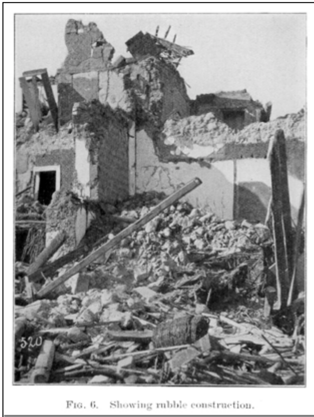
Figure 1. Photo-lithographic illustration of rubble construction destroyed by the 1908 Messina Earthquake. Frank A. Perret. "Report on the Messina Earthquake of 28, 1908." American Journal of Science 27.4 (1909): 327. Print.
