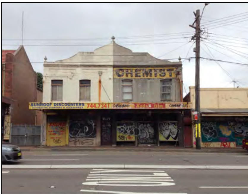
Figure 3: Abandoned Shops, Parramatta Road, Concord, 2015. Photo: Vanessa Berry.
